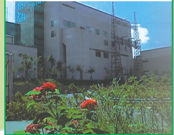
Hisnyu Co-Generation Plant
